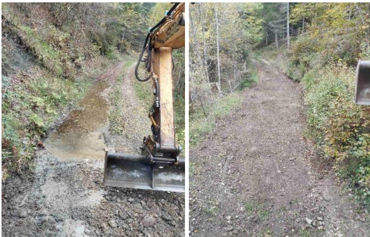
Figure 24. Pedological work on the arrangements of the gravel access road to the necropolis
