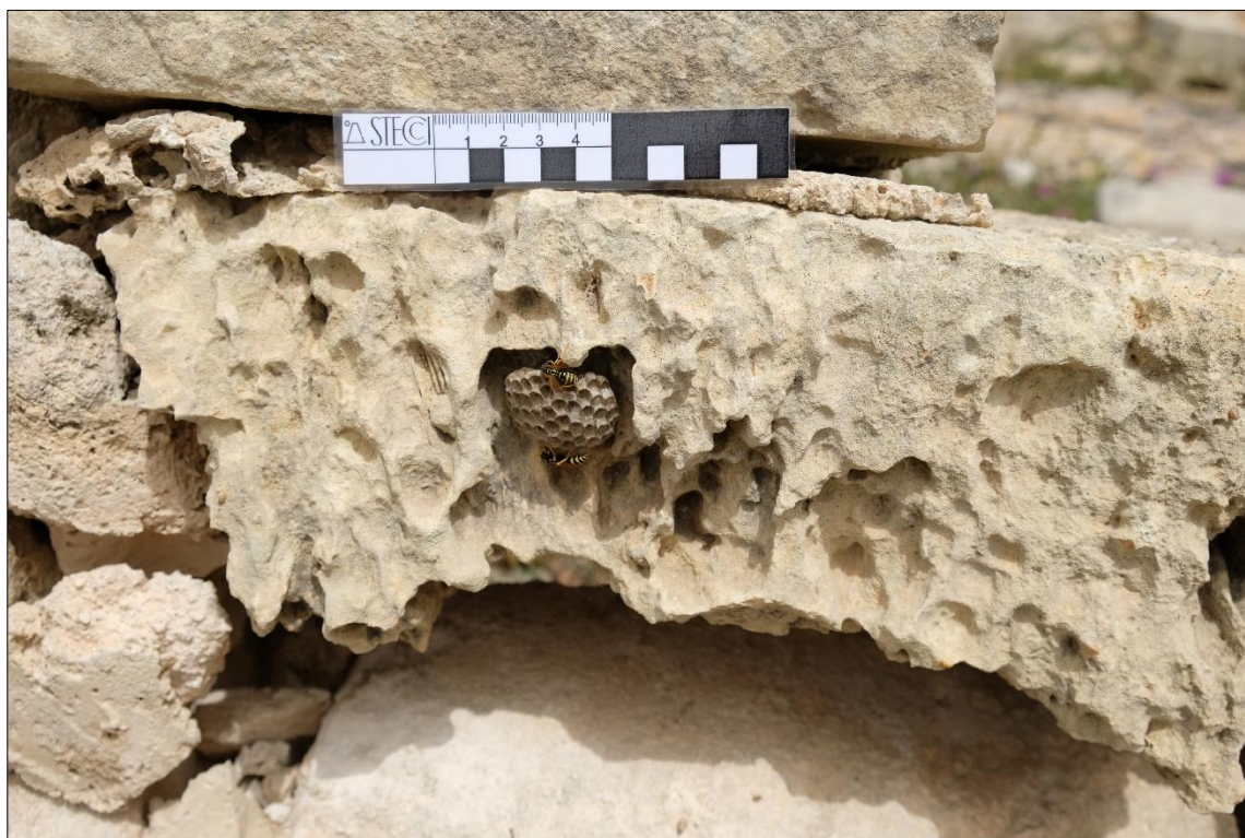
Fig. 7: Typical, “honeycomb” decay pattern is the result of the action of wind and salts on (mostly) porous limestones
